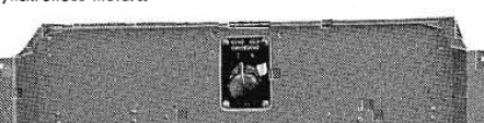
Sync Generator Switch, MI-26285. Used to switch outputs of either of two sync generators over to studio equipment. One selector for all 5 signals (horizontal, vertical, blanking, sync, and CRO sync).
