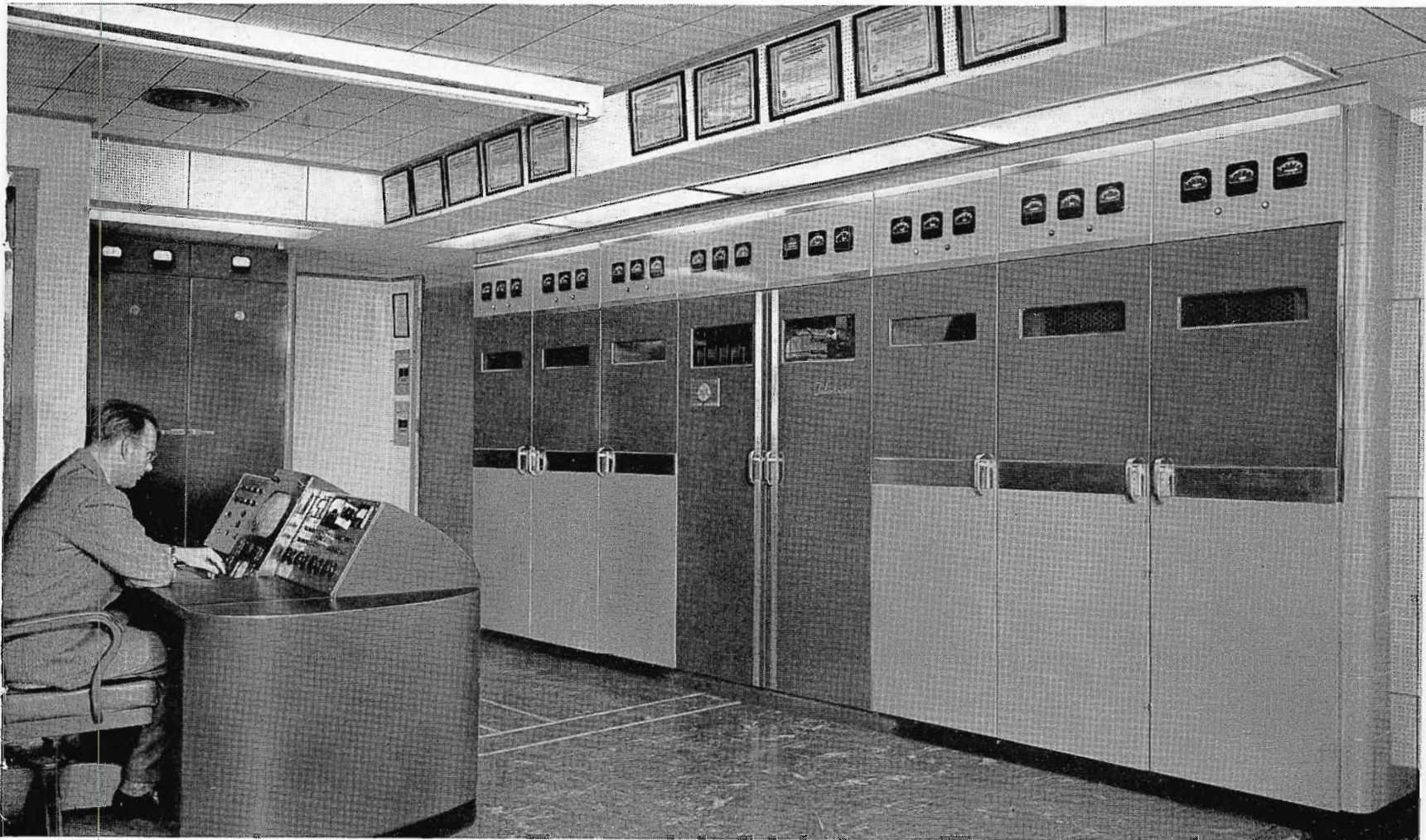
FIG. 3. Mr. Frank Vials, transmitter engineer of WAAM, seated at the console of the RCA TT-5A Television Transmitter. WAAM operates on Channel 13 with an effective 26.1 kw visual power and 13.8 kw aural power. The antenna is a six-section Super Turnstile.
