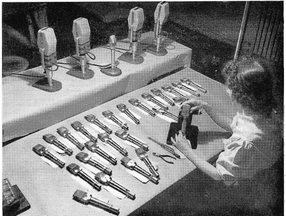
FIG. 2. The KB-2C Bantam Microphone (as shown in this production line photo) is much smaller than the popular Type 44-BX Velocity Microphone.
